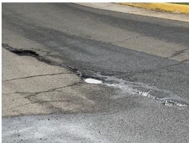
There are numerous potholes and cracks on the parking lot. It does not currently need to be milled and replaced, but the problem areas need to be patched and the entire surface resealed.
