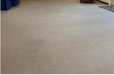
The carpeting in the vestibule and the office wing has reached the end of its useful life and needs to be replaced. It soils easily and cleaning can only do so much. It should be replaced with a long-lasting, high-traffic solution.
